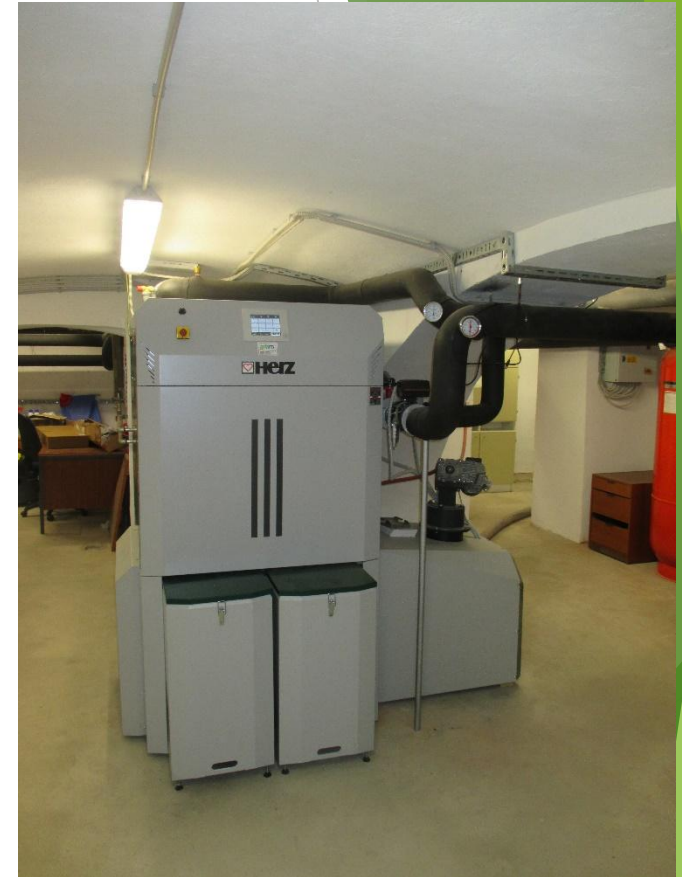
Herz Firematic 201 Type of fuel: wood pellets Nominal power: 201 kW Thermal efficiency: 89.7 %
